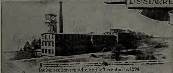
The two sections middle and left erected in 1894
